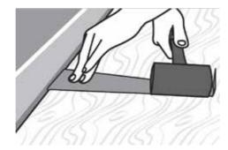
11. Once you have finished the final row cut the underlay to the height of the boards.
